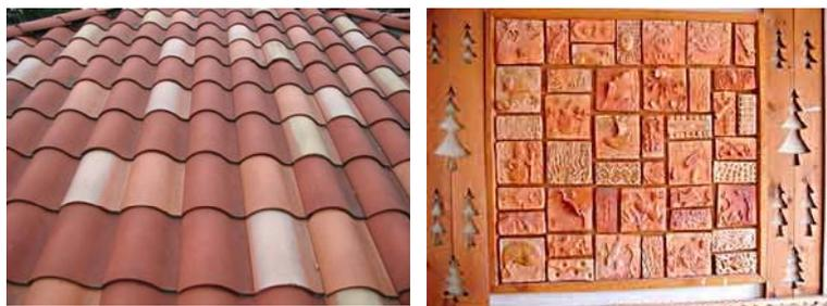
Tiles made using locally available clay should be encouraged rather than insisting only on the mangalore pattern clay tile for the purpose of roofing. Fibre reinforced clay tile is a good alternative material displaying high aesthetic performance and durability. The fibres could be any locally available agro waste.
