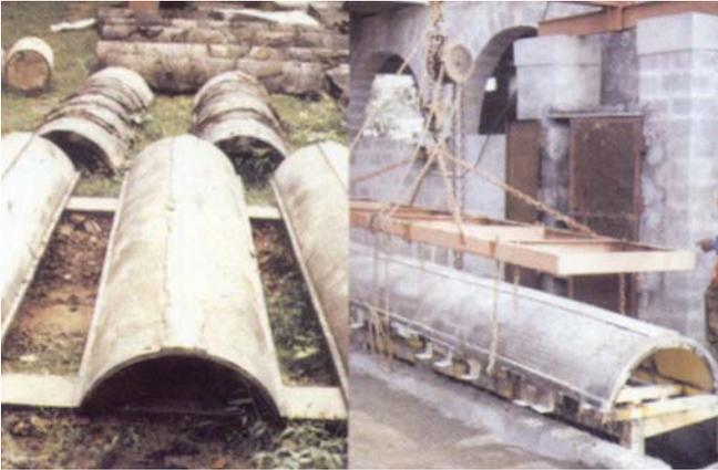
Precast in-situ thin ribbed slab made from precast/in-situ ribs provided at a spacing of 1.2 m with cast-in-situ RC flange. These can be used for floor/roof slab. As the ribbed slab is thin, roof treatment should be provided over the slab for better thermal insulation. It is cheaper and easy to construct in comparison to conventional cast-in-situ RCC slab.
