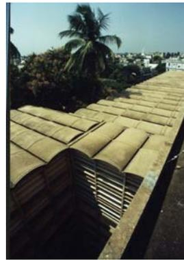
**Figure 11** Air gap acts as an insulation to reduce heat radiation from roof (Golconde, Pondecherri) Source: Bioclimatic Design, Undergraduate Thesis by Ravindra D. Gaekwad
