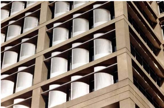
**Figure 20** Vertical light shelf; Source: [www.savannahtrims.com/images/Scane.jpg](http://www.savannahtrims.com/images/Scane.jpg)
