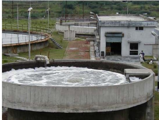
**Figure 4.** Aerobic treatment system, Source: Eco-housing training module.
